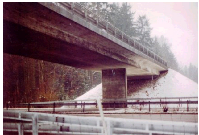
Z24 Bridge viewed from Bern-to-Zurich highway A1.
