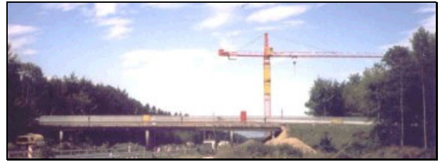
Z24 Bridge crosses Bern-to-Zurich Swiss highway A1.
