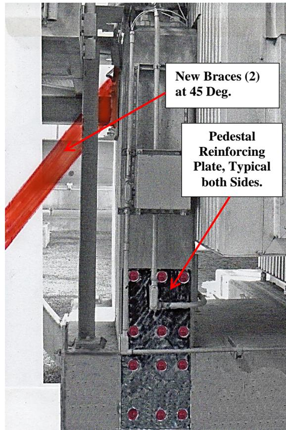
**Figure 39. Remove Existing Steel Braces and Install Two Braces at 45 Deg. Bolt Plate to Each Side of Pedestal & Concrete Foundation.**
