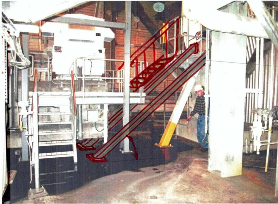
**Figure 41. FD Fan A OB Pedestal Bracing and Platform Access by Stairs Modification.**
